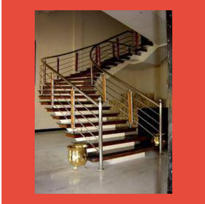
Stainless Steel Railing
